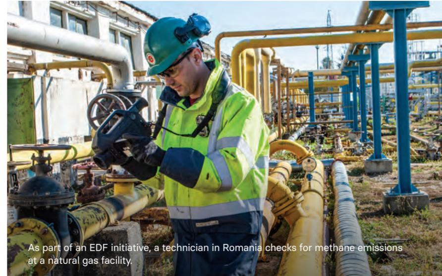
As part of an EDF initiative, a technician in Romania checks for methane emissions at a natural gas facility.
